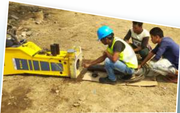
Breaker Service Camp
